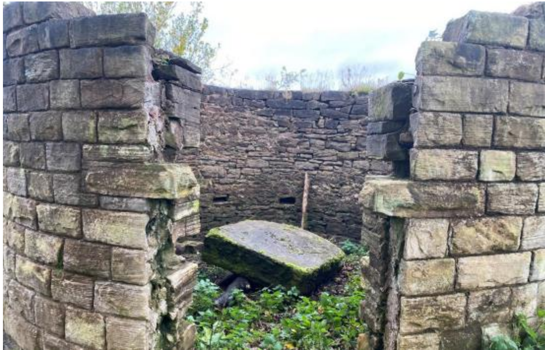
Photo 6: Derelict building to be converted
