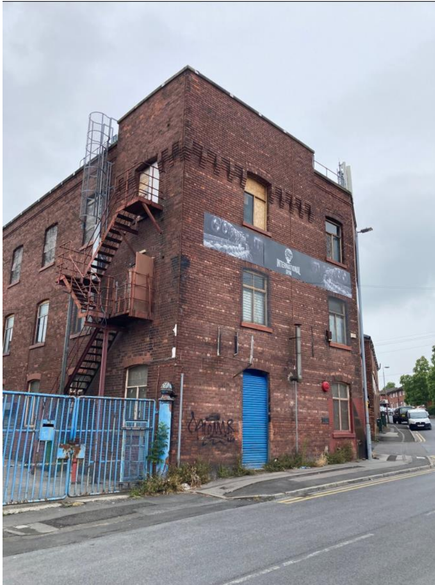
Photo 3: View of side of building, facing wall of neighbouring industrial use
