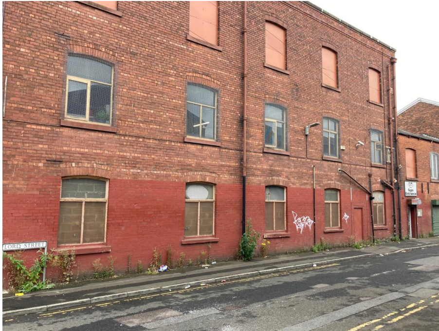
Photo 5: View of side of building viewed from Lord Street
